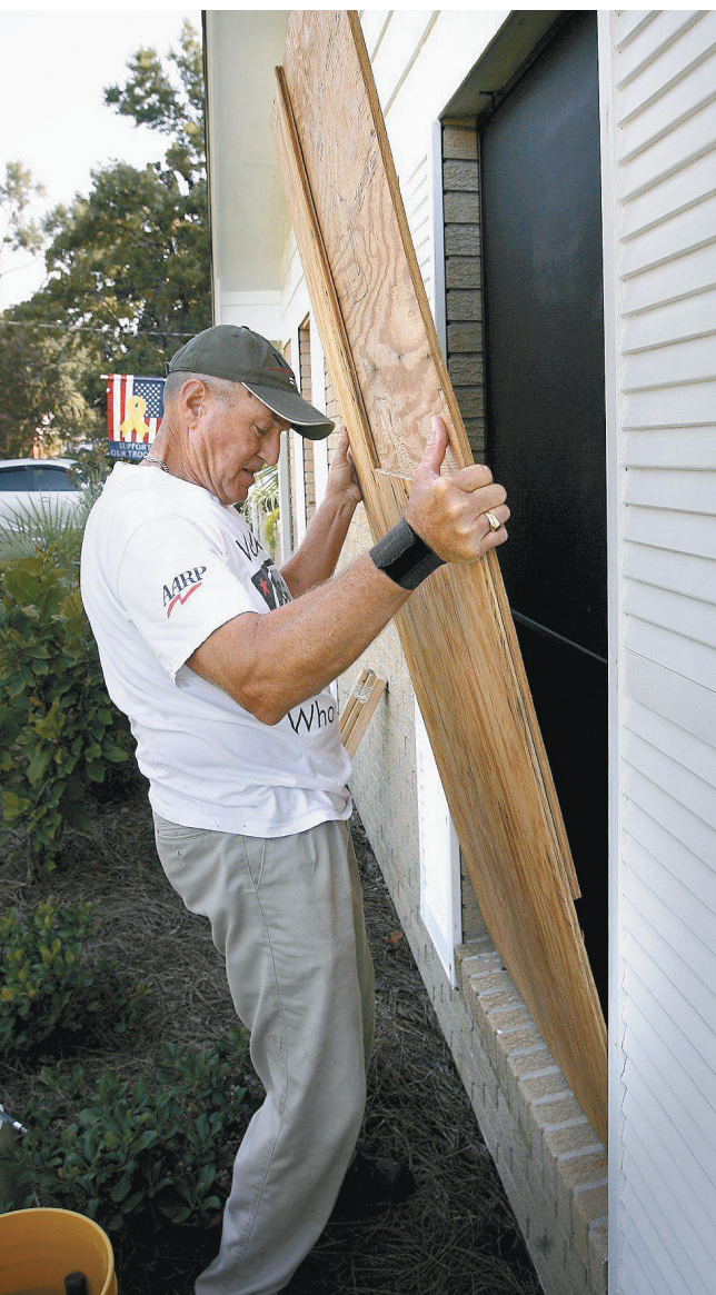
SUN HERALD FILE PHOTO — Plywood sheet, in quarter or half-inch thickness, offers the best protection for windows from limbs and other flying debris during a hurricane.
